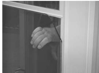
**Step 2:** Move operating glass insert into the closed position.
