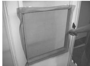
**Step 7:** Roll the screen spline and screen into the screen channel along bottom.
