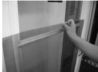
**Step 4:** Locate the approximate middle of the screen spline length and using the cupped wheel on the screen roller, push the screen fabric with screen spline into the middle of the top screen channel. Roll the screen fabric with screen spline into the entire length of the top channel.
