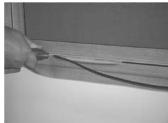
**Step 8:** Carefully cut the screen spline and push the ends into the screen channel anywhere along the bottom screen channel.
