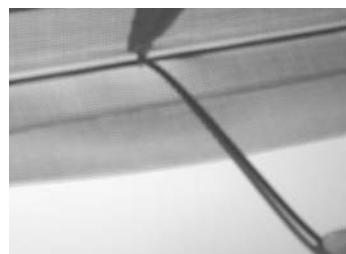
**Step 9:** Carefully trim the screen fabric using a utility knife and running it along the outside edge of the screen channel.
