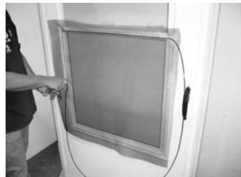
**Step 6:** Roll the screen spline and screen fabric into the screen channel along the right-hand side while pulling slightly on the lower corner of the screen fabric to prevent wrinkles.
