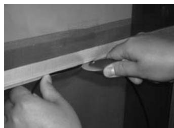
**Step 5:** Roll the screen spline and screen fabric into the screen channel along the left-hand side.
