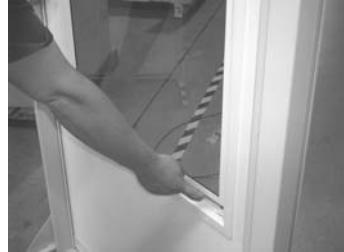
**Step 3:** Tape the screen fabric to the glass at the top, about 1" above the meeting rail, to allow it to hang centered over the screen opening with the fabric grids align with the frame. The screen fabric should overlap the screen frame on all sides when complete.
